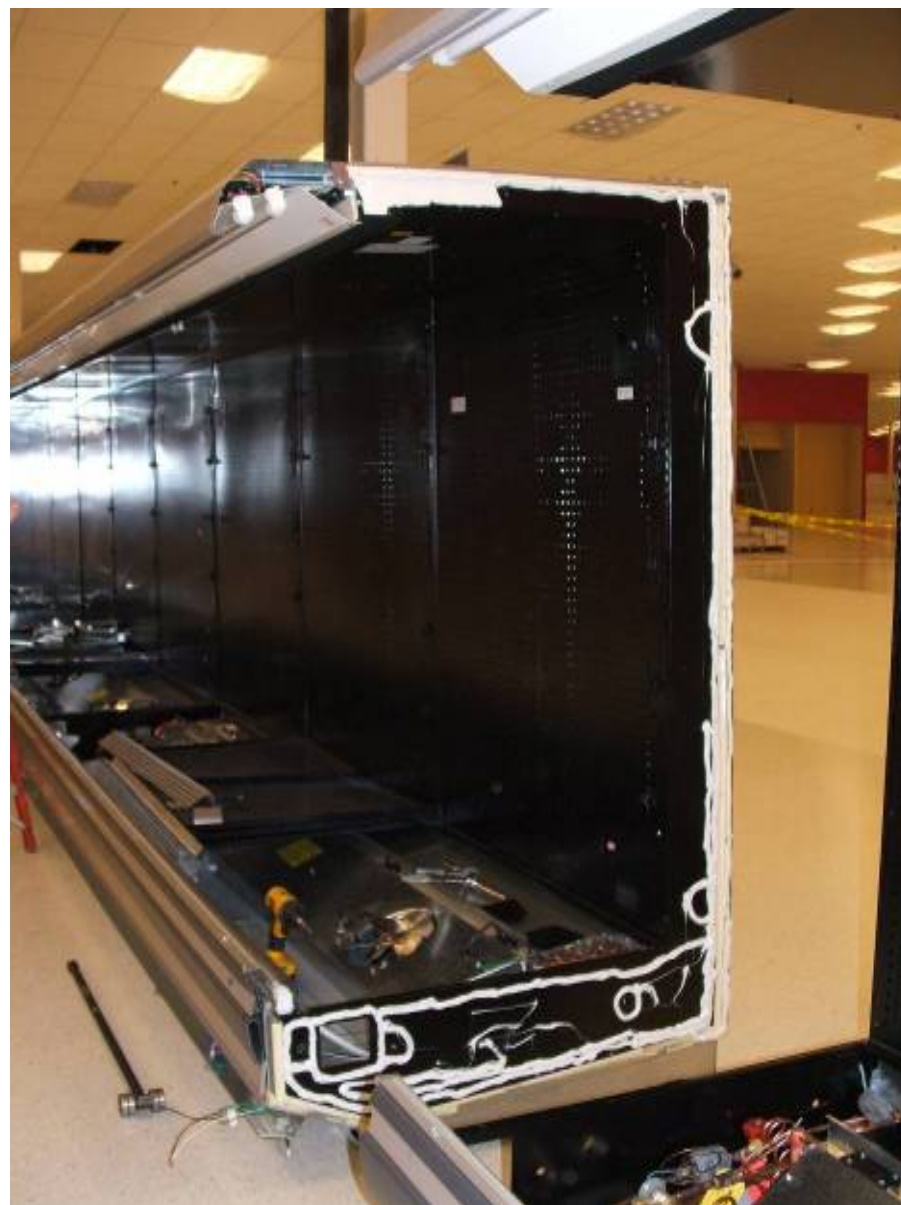
Case to Case Sealant Application
