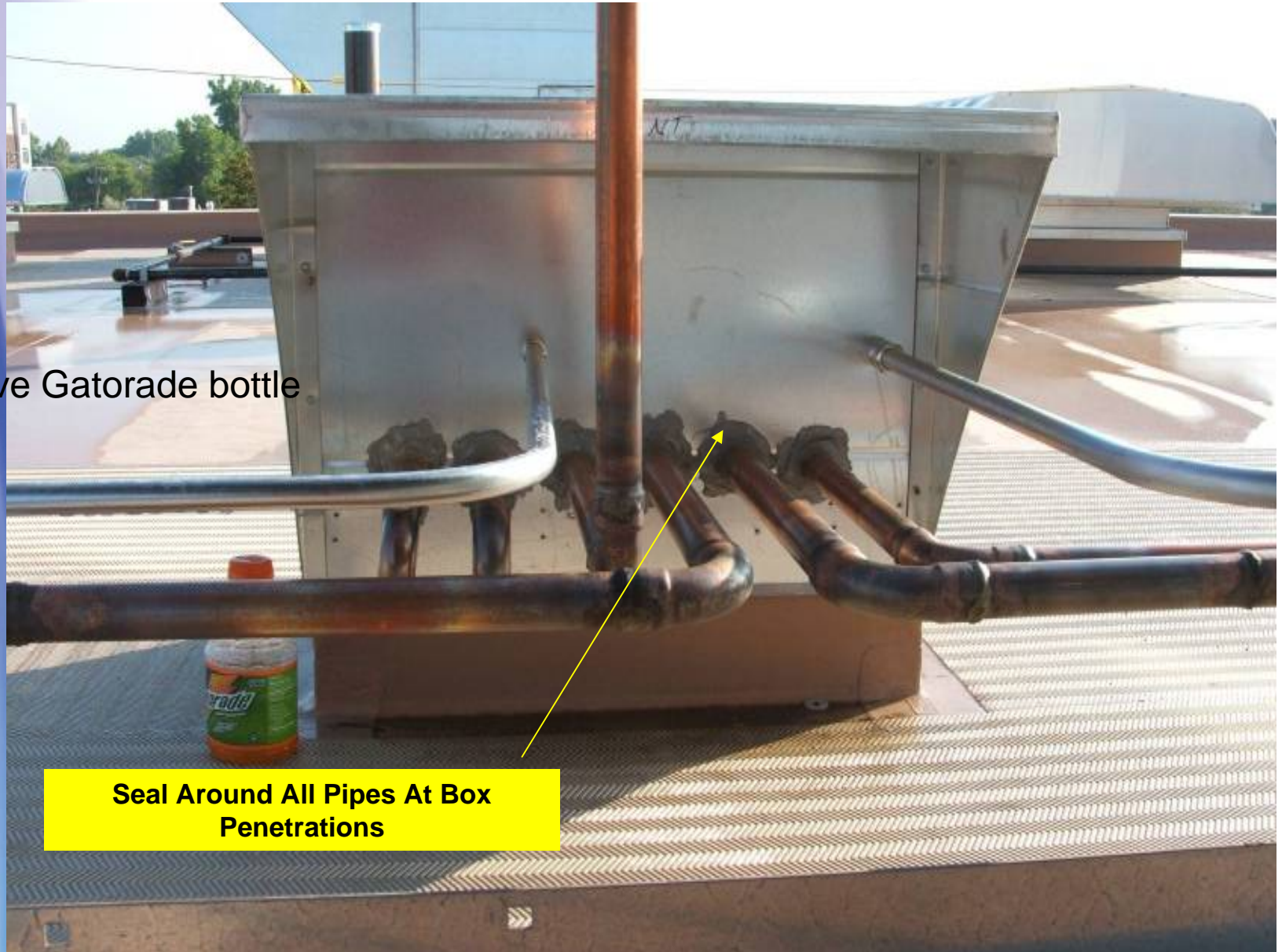
Condenser Pipe Support Detail
