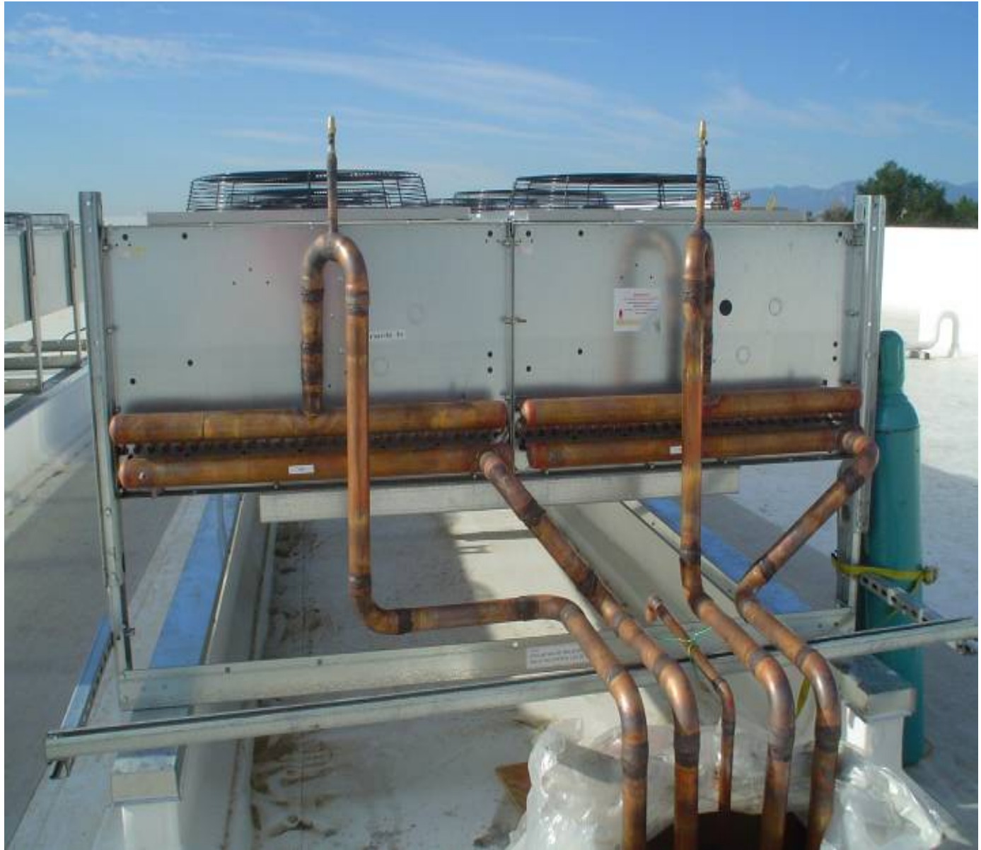
Condenser Pipe Support Detail
