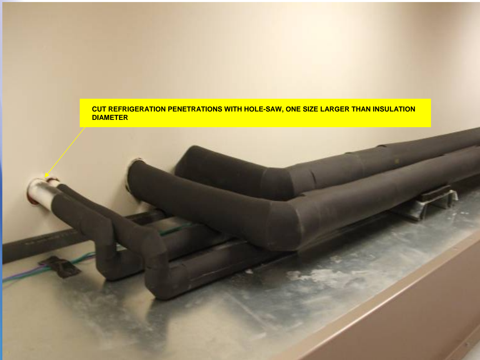
Refrigerant Piping For Sales Floor Cases @ Wall
