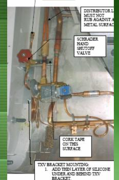
USE EXISTING SCREW IN PIPE CHASE TO LOCATE AND MOUNT
